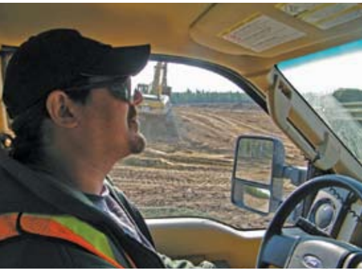
KDFN citizen, Chris Trociuk, is working as a Project Inspector at the Whistle Bend Subdivision.
