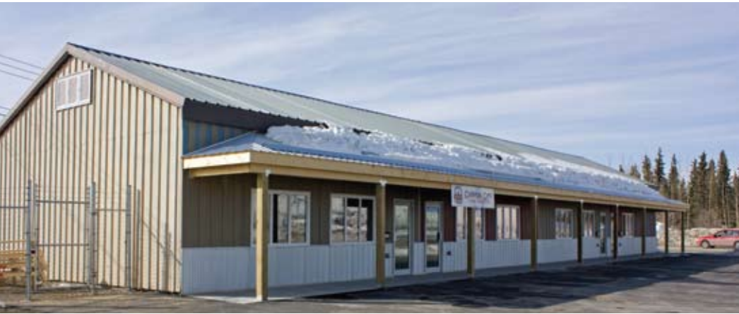
The new offices of Canyon City Construction are on the corner of Tlingit and Platinum. The KDFN company is a for-profit business that employs qualified citizens whenever possible.
